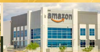
Amazon Data Center
